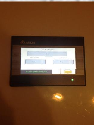
level by regulating soil moisture in the greenhouse in the database stores all the parameters. You can use any analogue sensor system that collects information. Automation system can be controlled via the internet. At the same time the system has internet information system on the web. Automatic irrigation system project, the automation of electronic systems and software control program, made greenhouse prototype has been tested and was found to be applicable.
